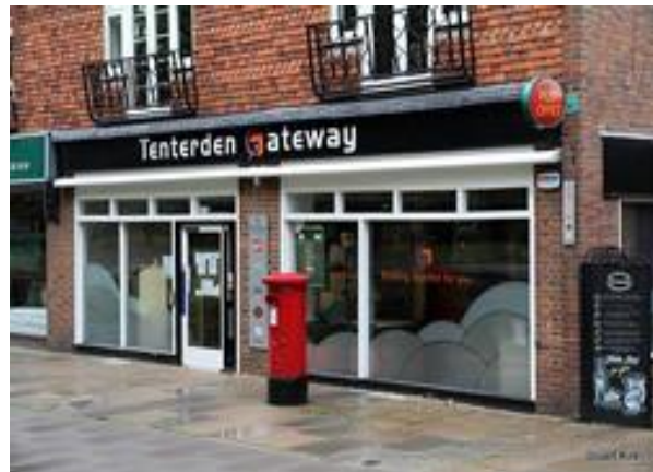
Combined Post Office, Library & Drop-in Centre
